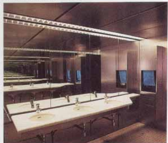
Stainless steel interior cladding.
