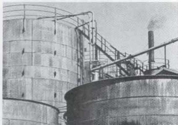
Rivetted stainless steel nitric acid tanks at ICI Ltd, Billingham 1929.
